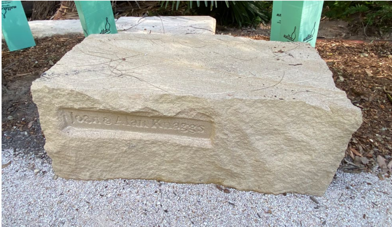
Figure 6: Engraved Grade 1 sandstone block (“logs”) 1000 x 500 x 500. the area behind the lettering is dressed.
