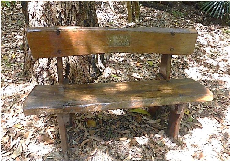
Figure 3: An existing example of the rustic timber bench seat with no arms (Type A2). It is considered that these seats would need less future maintenance as there are less areas for water to collect and cause rot.
